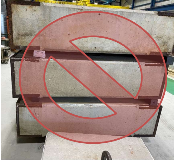
Shield blocks stacked in multiple layers using non-rated plastic lumber – not acceptable
